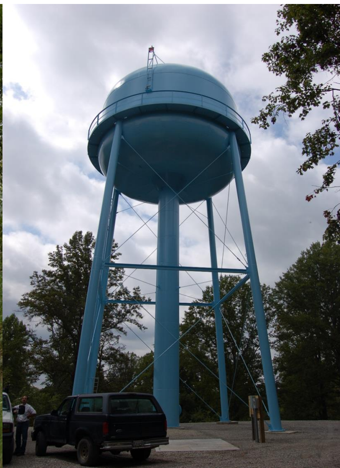
Left: New Rose Ridge water tower with the old storage tank in the foreground. Right: New 200,000-gallon Rose Ridge water tower. Photos courtesy of Leman Kendrick.
