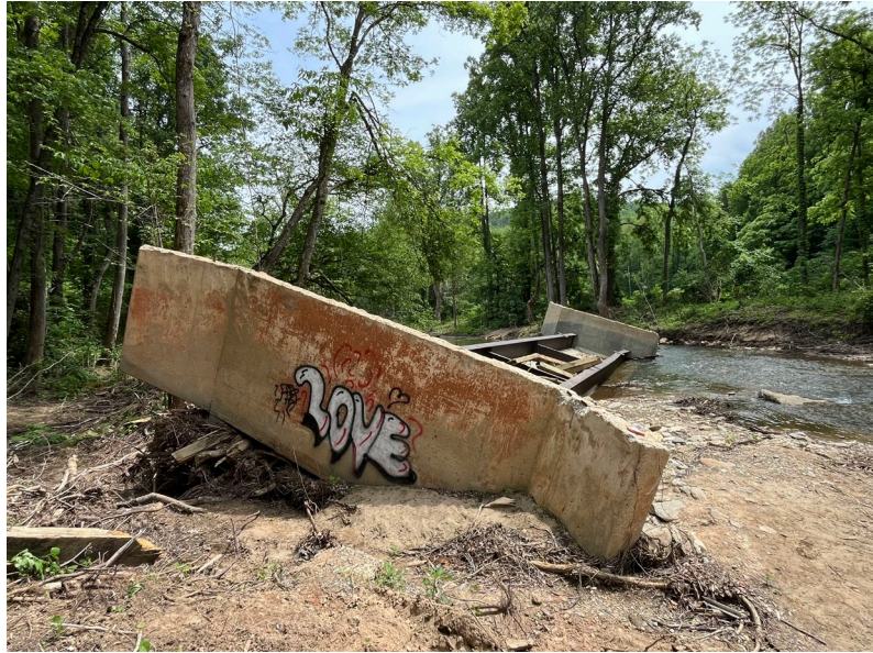
Photo: Vehicular bridge within the Pisgah National Forest near Old Fort, NC completely upended by flood waters. This damage has cut off access to some of the area's most popular hiking and mountain biking trails.
